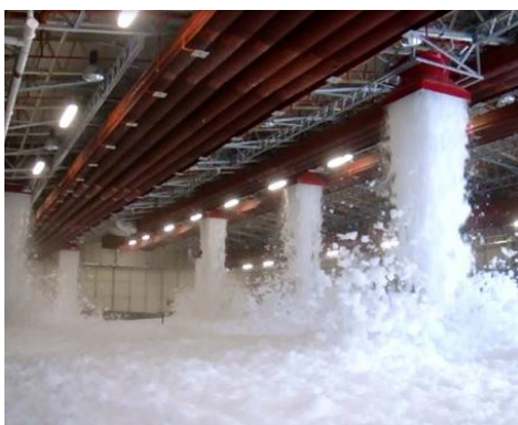
Figure 1 Foam sprinkler system [3]
