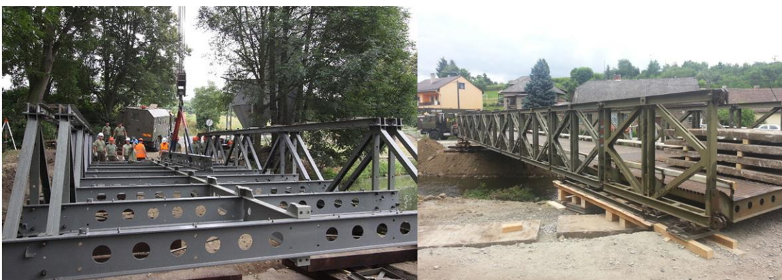
Figure 2: Assembling of the bridges
