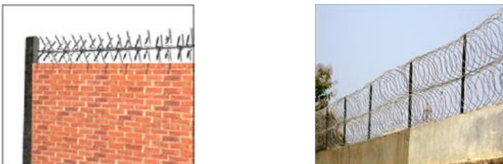
Figure 14 a) Higher barriers made of movable centres, b) The Concertina wire higher barriers
