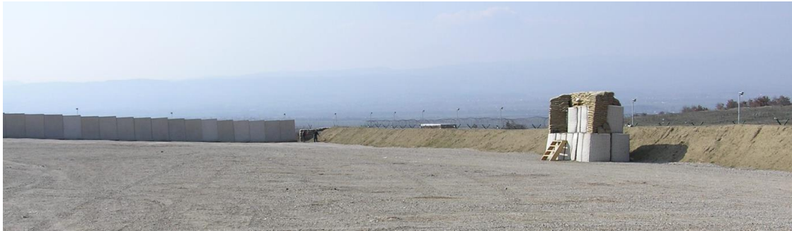
Figure 1 Barrier protection – Protecting earth embankment and T-wall. The Base Šajkovac protection in mission KFOR
