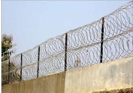
Figure 4 a) Razor wire on the top of barrier, b) The razor wire in detail
