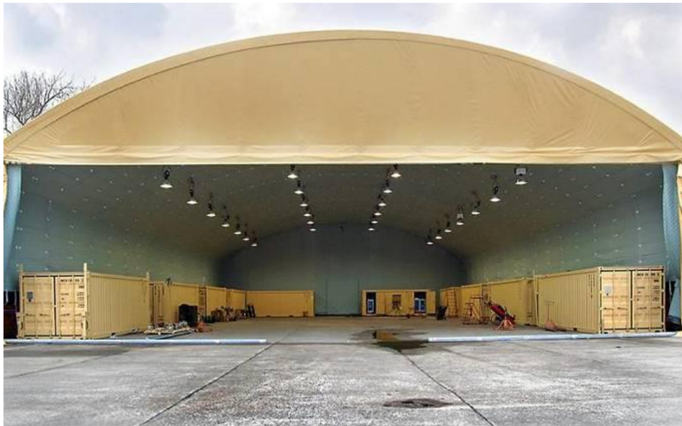
Figure 4 Hall designed for helicopter repair [2]
